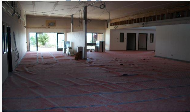
View Looking Into Building I from West Hallway
